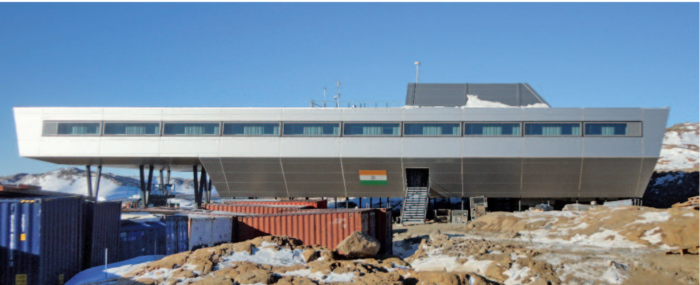
India's Bharati Research Station just prior to completion: insulation panels of zinc-magnesium coated steel sheet with organic coating fulfil the most demanding requirements, even at temperatures down to minus 45 °C.
