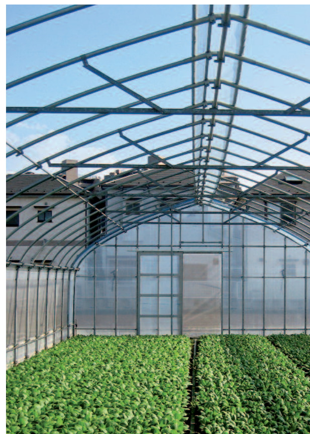
Greenhouse: profiles of zinc-magnesium coated steel sheet form the supporting construction
