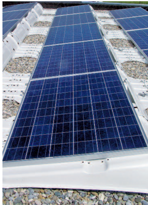
Frames made from organic coated zinc-magnesium steel sheet for mounting photovoltaic elements
