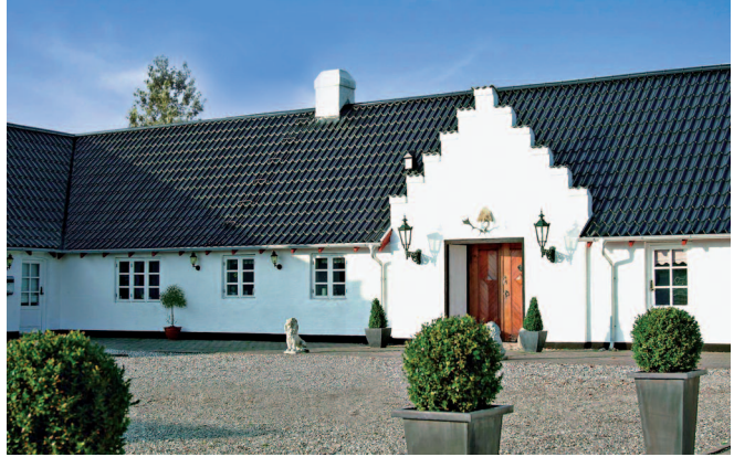
Manor house in Denmark with anthracite steel pantiles
